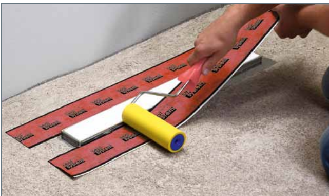
Seal System adhesive tape: the butyl adhesive tape is a self-adhesive sealant and ensures a water-tight bond between the flange and the screed.
