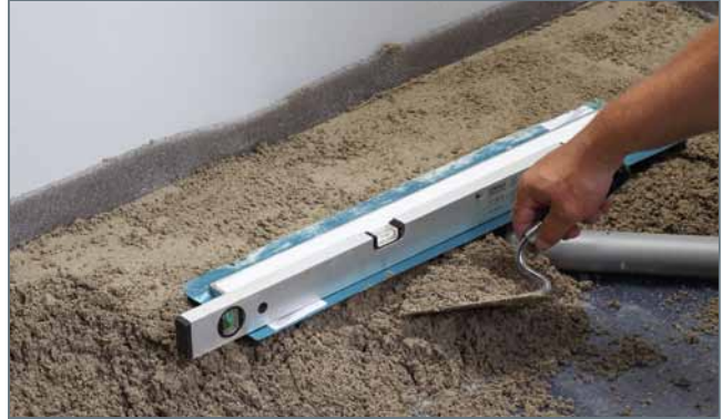
Complete underfilling with screed produces stable anchoring of the channel body and outlet with the unfinished floor.
