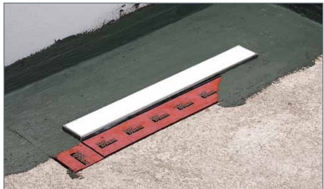
The final step before tiling is the application of the composite seal.
